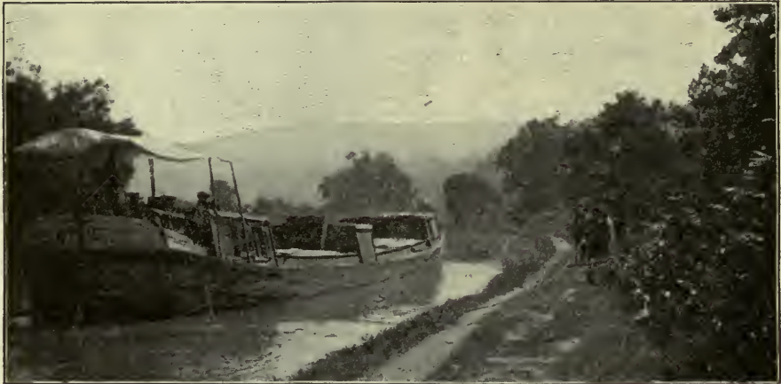
FIG. 51. — A canal boat in a canal dug around rapids in a river.
